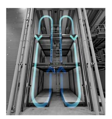
Air flowing through the evaporator is circulated into the space between the pallets and the room walls. In conjunction with our sealing system, we can ensure equal ripening throughout the room. Optionally, your system can be fitted with a reversible air circulation system for guaranteed results.
