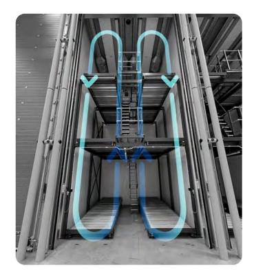
Air flowing through the evaporator is circulated into the space between the pallets and the room walls. In conjunction with our sealing system, we can ensure equal ripening throughout the room. Optionally, your system can be fitted with a reversible air circulation system for guaranteed results.
